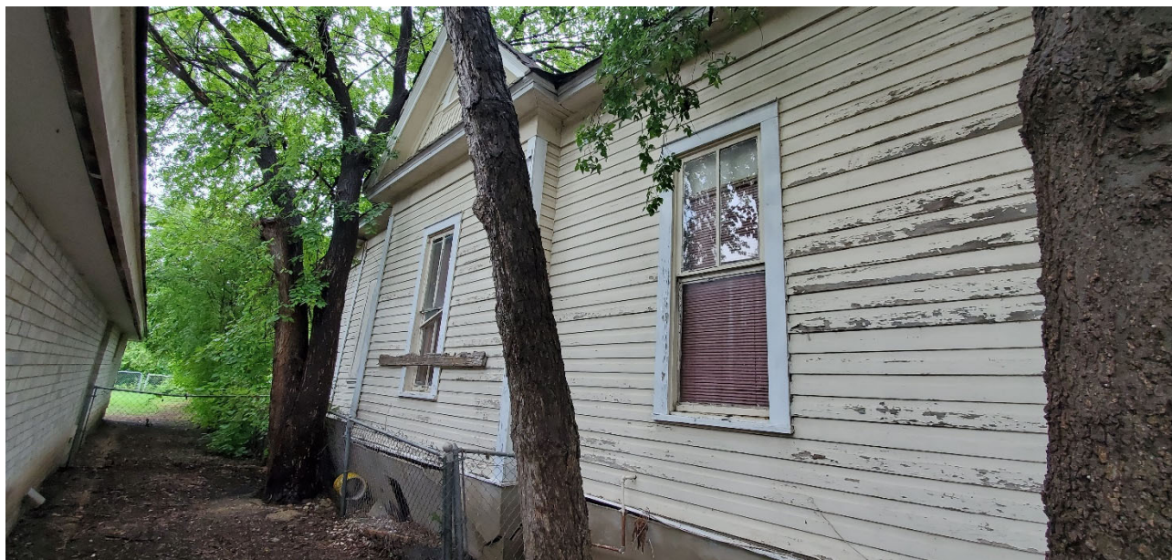
West elevation with two-over-two windows.
