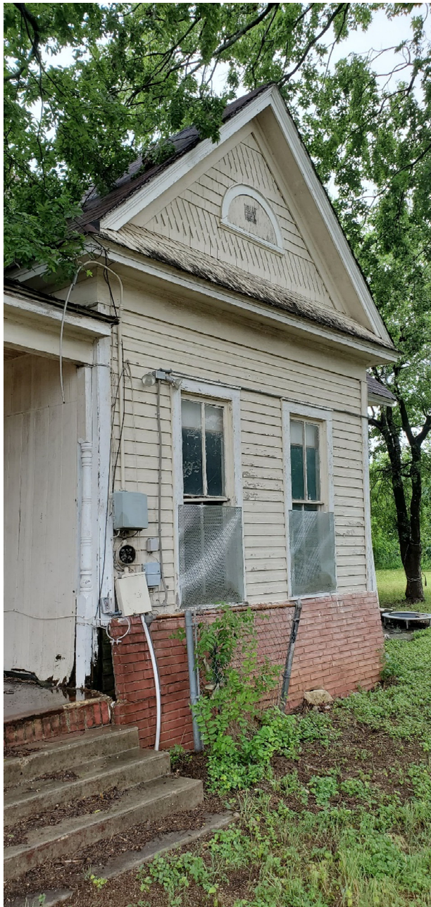
East elevation details: Gable and historic turned wood pilaster.
