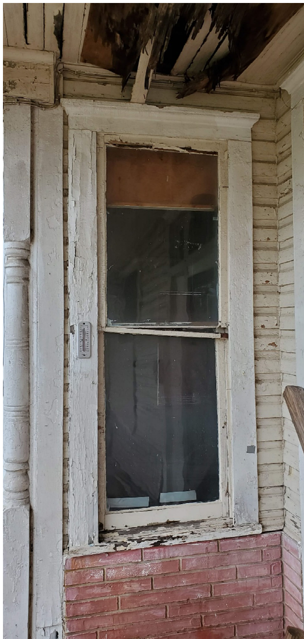
One-over-one and two-over-two wood windows on the porch.
